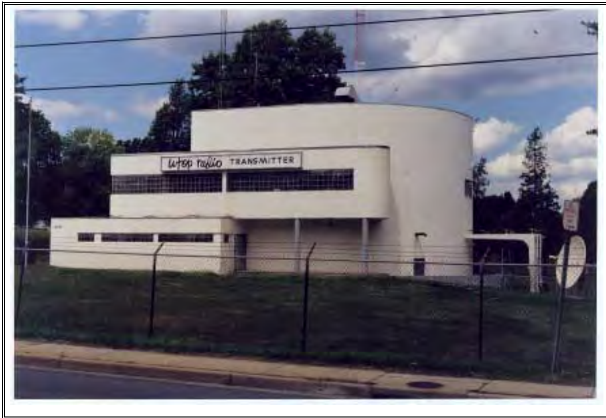
Plate 2: "Streamlined" building (WTOP Radio, 2021 University Blvd., Wheaton)
