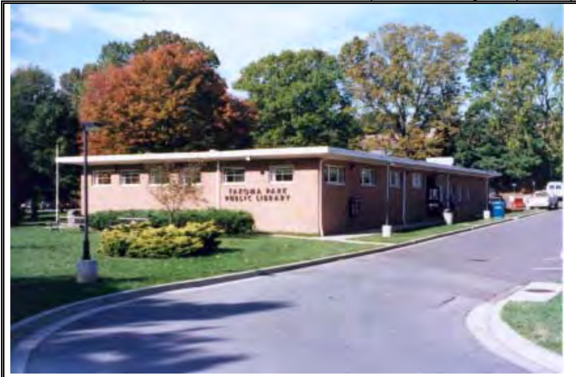
Plate 33: Library (Maple Avenue, Takoma Park, Montgomery County)
