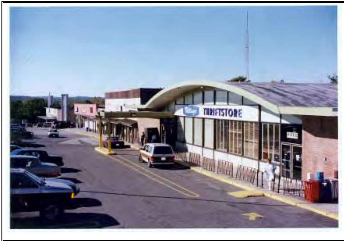
Plate 3: Standard shopping center (Village Thrift Shopping Center, 5600 Annapolis Blvd., Bladensburg)
