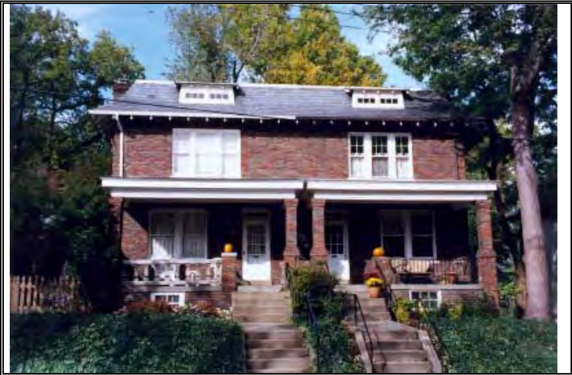
Plate 21: Double House/Duplex (3637-3639 Jenifer Street, Washington, D.C.)
