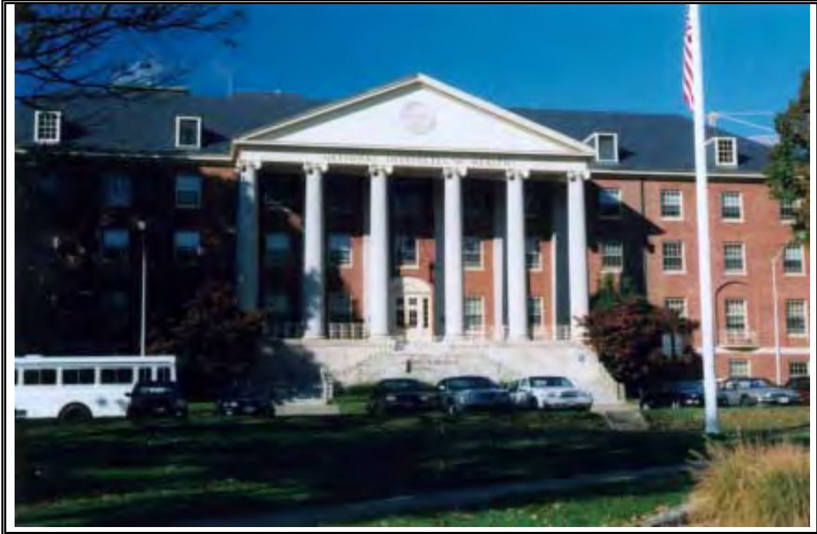
Plate 38: Hospitals (National Institutes of Health, Building #1, Bethesda, Montgomery County)
