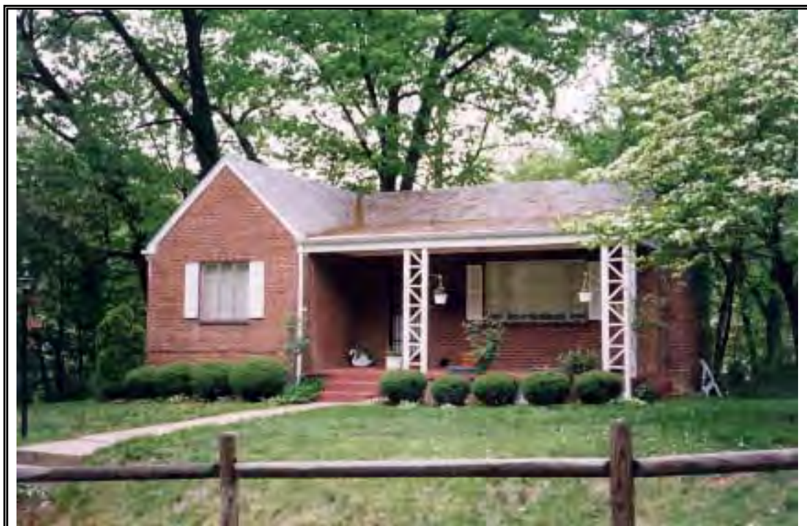
Plate 19: Minimal Traditional House (9800 Grayson Avenue, Four Corners, Montgomery County)
