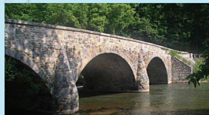
Booth's Mill Bridge (MD 68 over Antietam Creek) 1833, Boonsboro, Washington County 7
