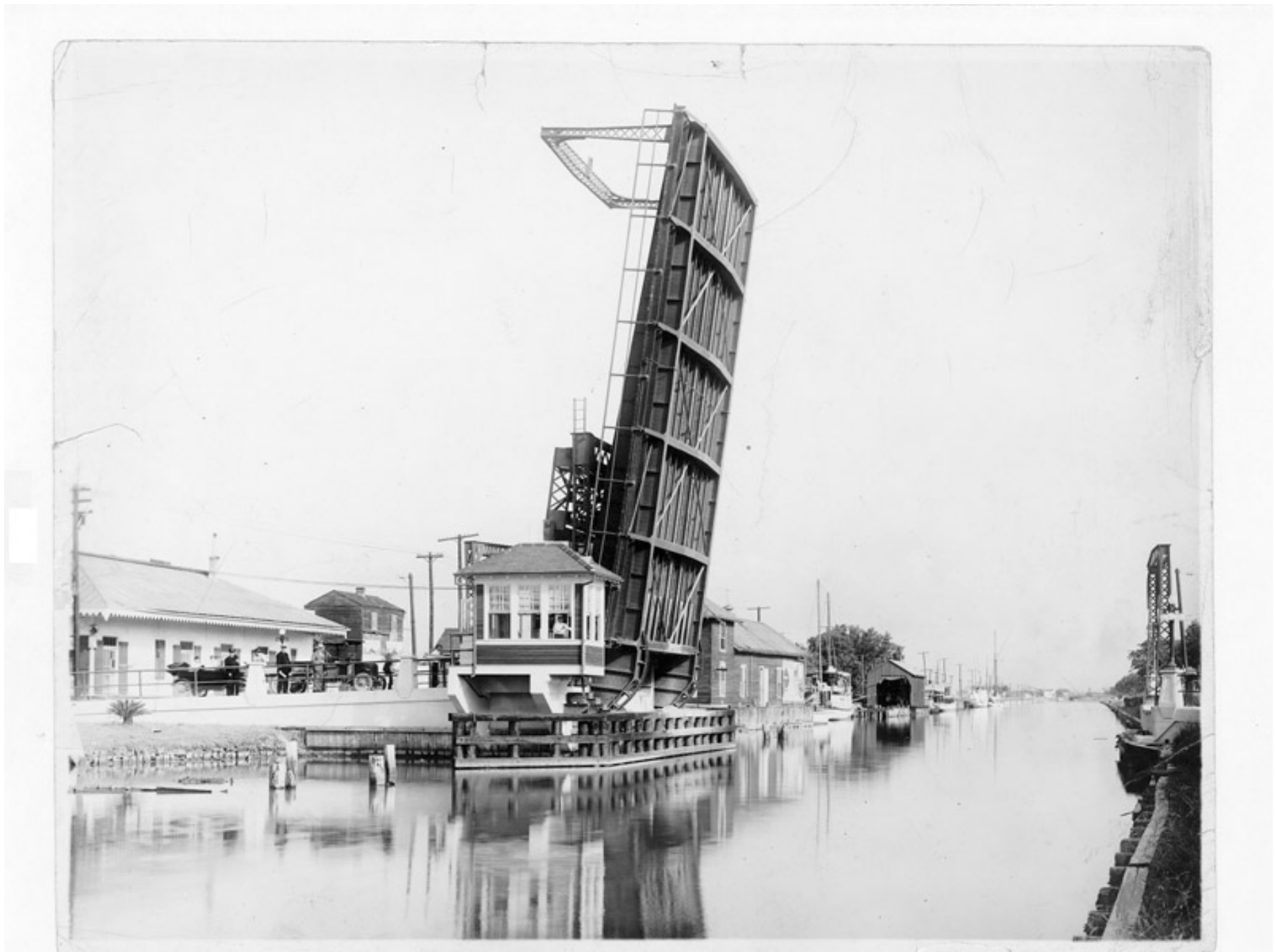
PLATE 8: Typical Single-Leaf Bascule Movable Bridge: Bridge at Kent Narrows
