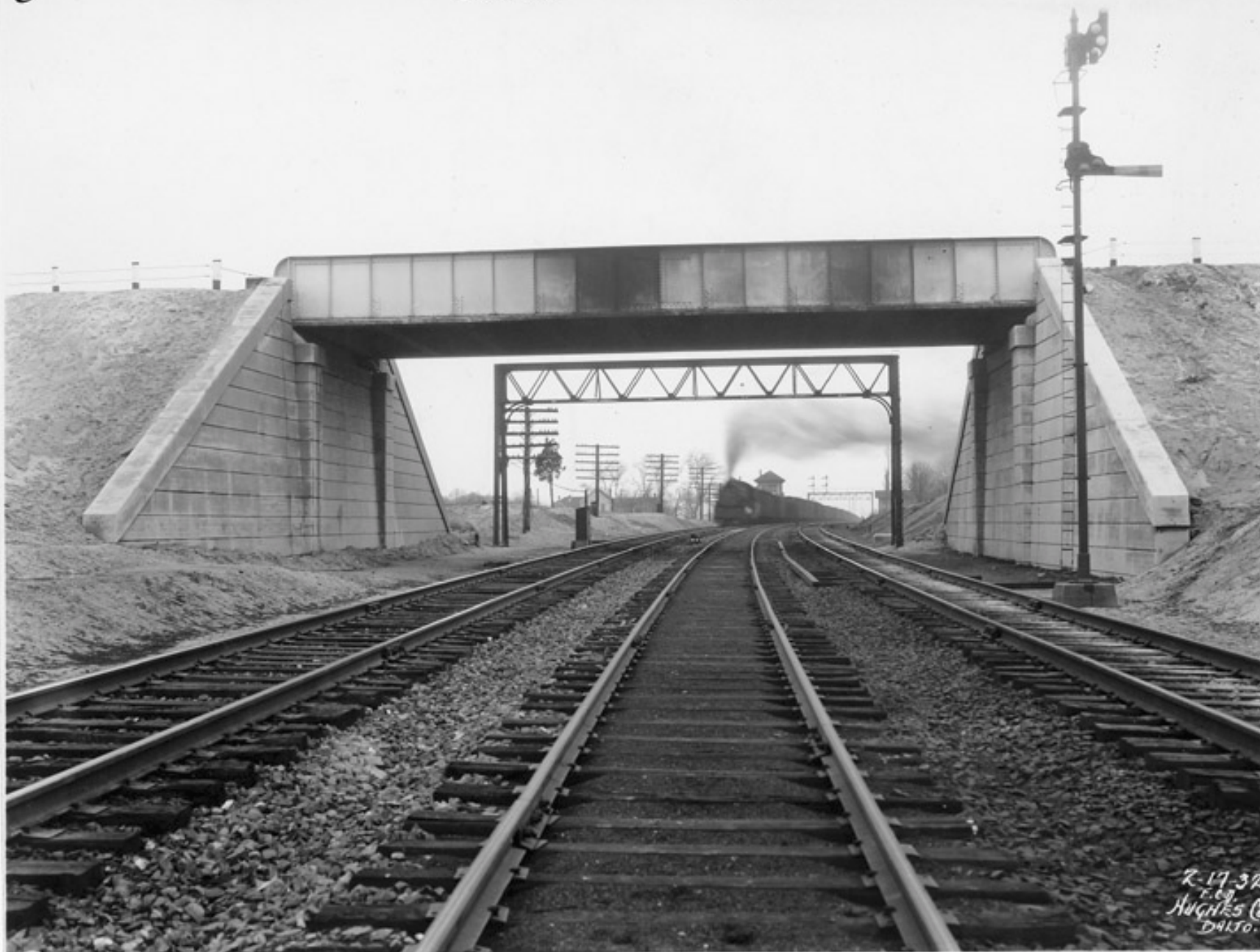
PLATE 10: Typical Metal Plate Girder (Through) Bridge: Crossing Railroad Tracks at Severn
