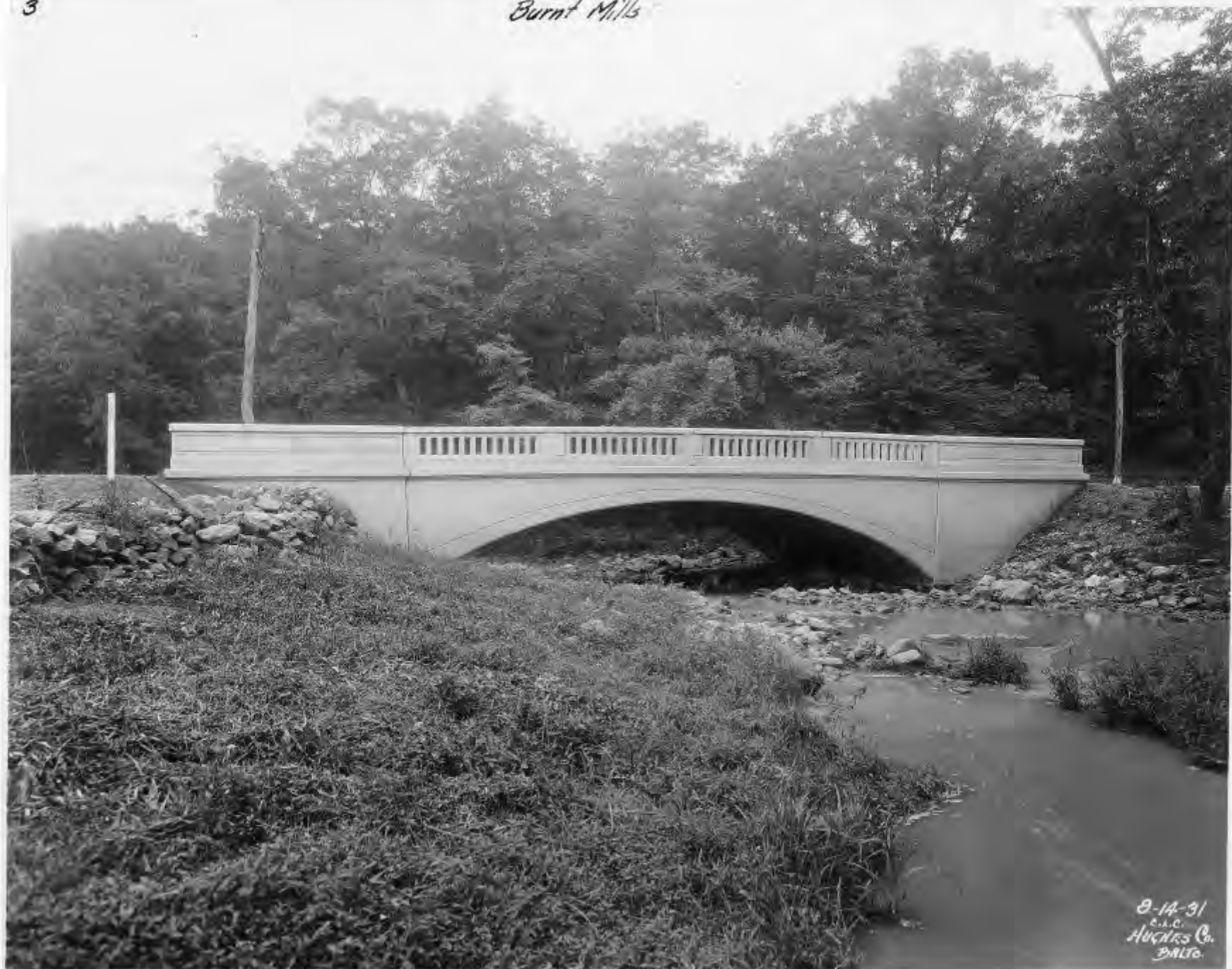
PLATE 13: Typical Concrete Closed Spandrel Arch Bridge: Bridge at Burnt Mills
