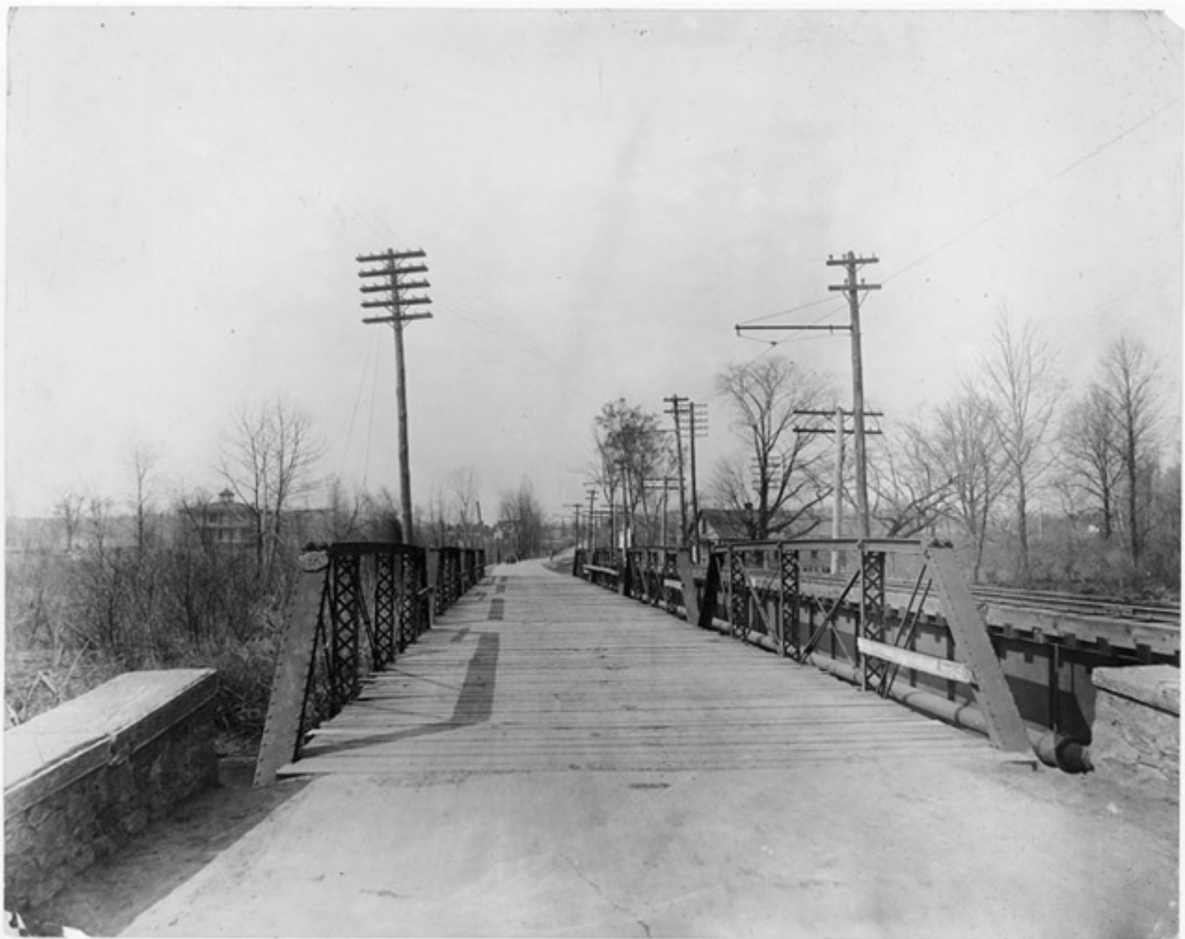
PLATE 6: Typical Metal Multiple-Span Pratt Pony Truss Bridge: Bridge Crossing Winter's Run at Edgewood
