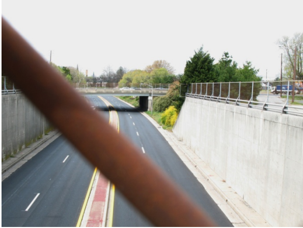
Figure 13: US 50 looking west towards Baptist Street, Salisbury (photo by Carol Ebright, SHA, 2007)
