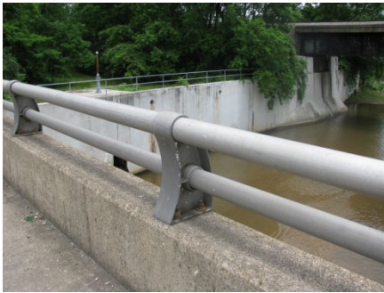
Two-strand aluminum railing and concrete parapet
