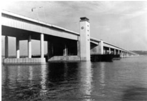
Figure 16: Woodrow Wilson Memorial Bridge, I-495 over the Potomac, looking east toward Maryland (SHA Photo Archive)
