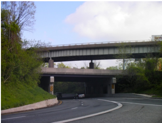
Multiple Fabricated Girders/Stringer Multi-Beam/Girder (SHA Bridge No. 0210100, MD 2 over US 50, Annapolis, MD). This is an example of multiple girders welded together.
