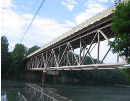
Steel Deck Truss (SHA Bridge No. 0604900, MD 26 over Liberty Reservoir, Carroll County, MD)
