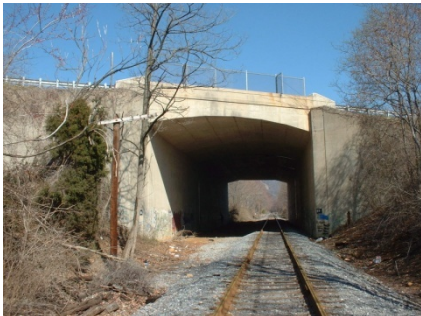
Concrete Rigid Frame (SHA Bridge No. 1010800, US 15 over Midland Railroad, Frederick County, MD)
