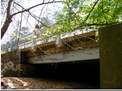
Concrete Encased Steel Beam, SHA Bridge No. 0205000, MD 176 over Piney Run, Anne Arundel County, MD
