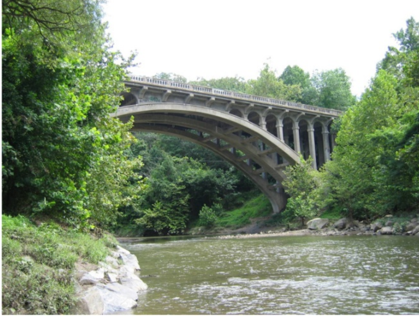
Figure 1: US 40 over the Patapsco River, Baltimore County (Photograph by Melissa Blair, SHA, 2007)
