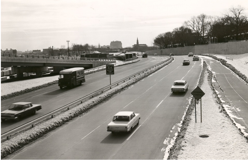
Figure 14: Jones Falls Expressway looking south near North Avenue (SHA Photo Archive)
