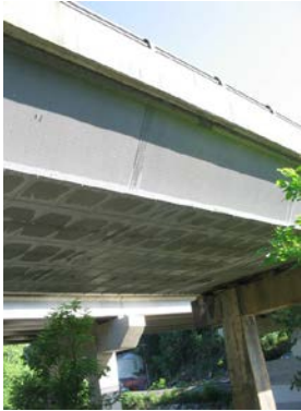
Aluminum Box Beam Bridge (SHA Bridge No. 1304600, Old MD 32 over River Road, CSX, and south Branch of Patapsco River, near Sykesville, Carroll County, MD)
