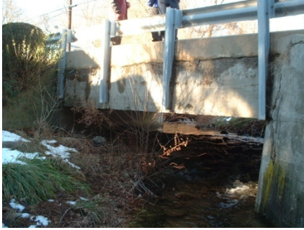
Tee Beam (SHA Bridge No. 1000600, MD 806A over High Run, Frederick County, MD)
