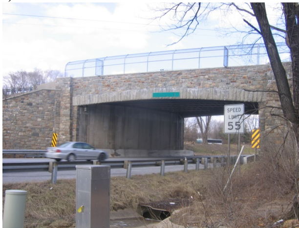
Figure 6: MD 168 over MD 295 Northbound, SHA Bridge No. 0201200 constructed in 1949 (photo by Anne Bruder, SHA, 2009)
