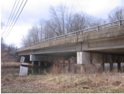
Concrete Box Beam Bridge (SHA Bridge No. 0802200, MD 225 over Mattawoman Creek, Charles County, MD)
