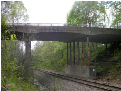
Concrete slab bridge (SHA Bridge No. 1611200, MD 381 over Norfolk Southern Railroad, Prince George's County, MD) --the sections at the piers are haunched or deeper in order to accommodate the stress of the traffic on the deck above.
