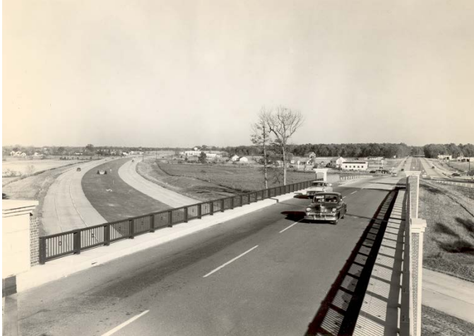
Figure 7: US 50 Westbound of US 301 Northbound, Queen Anne's County, MD (Source: SHA Photo Archive)
