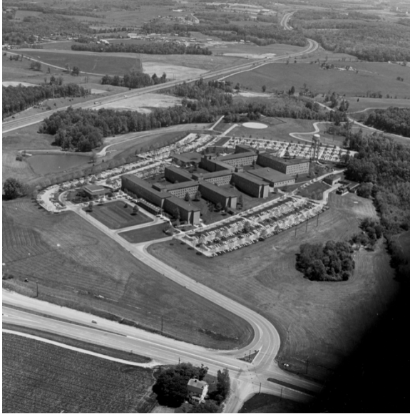
Figure 12: Atomic Energy Commission complex, Germantown, Montgomery County looking southeast at MD 118 (foreground) and US 240 (now I-270) in background 55
