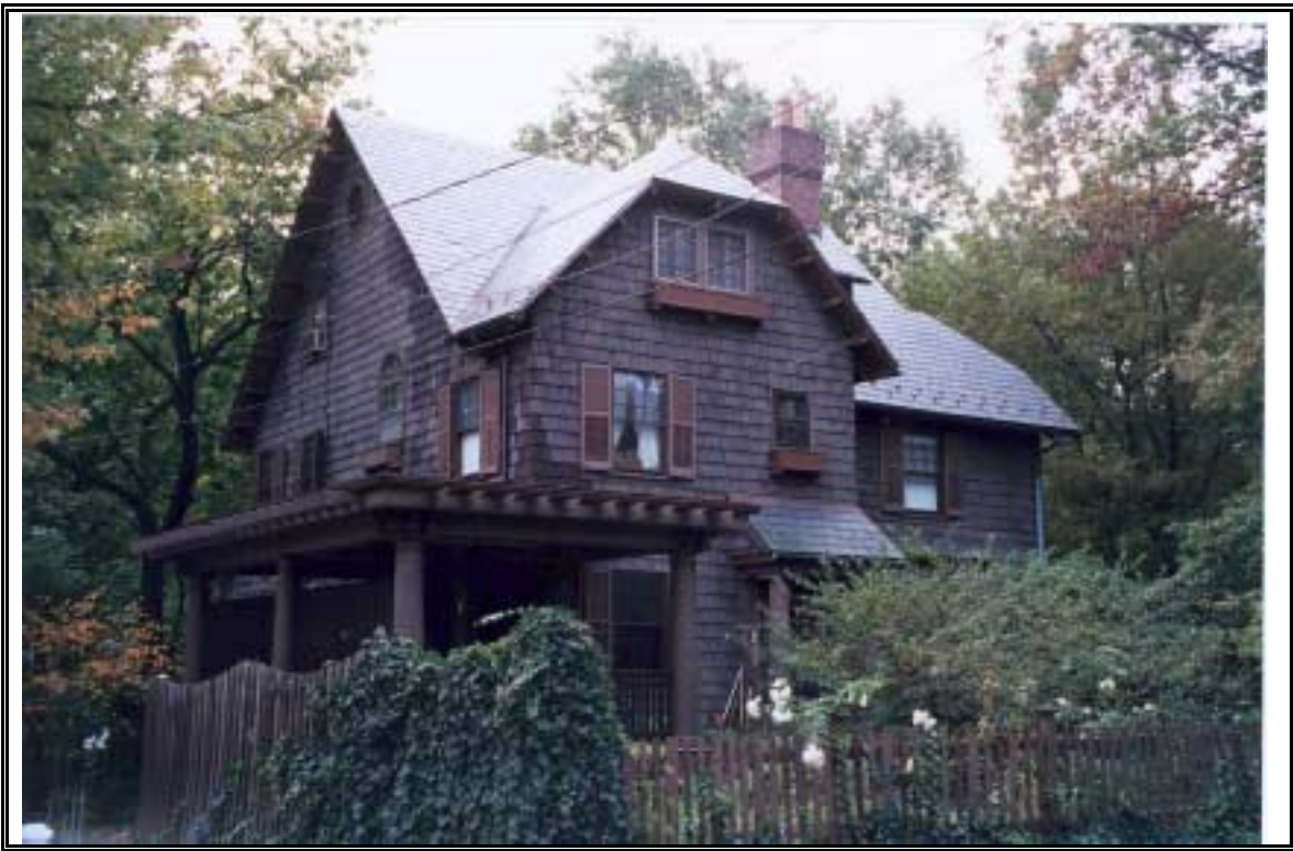
Plate 10: Shingle (3300 block of Newark Avenue, Cleveland Park, Washington, D.C.)
