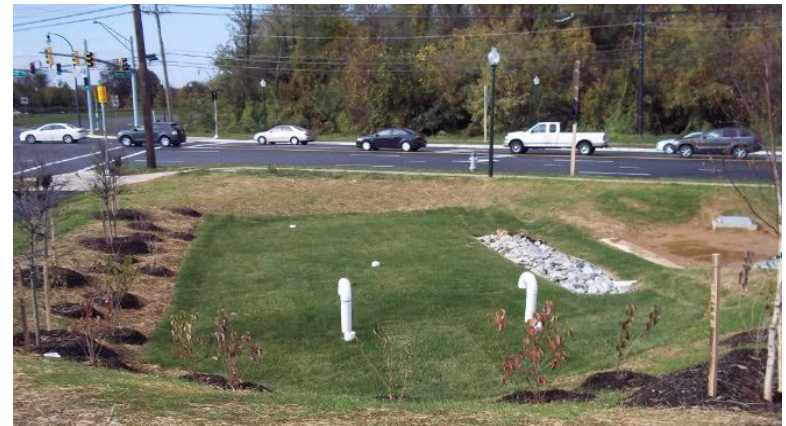
Figure 1-9: Surface Sand Filter along MD 355 in Montgomery County
