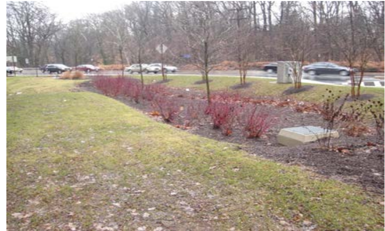
Figure 1-10: Bioretention Facility at MD 139 in Baltimore County
