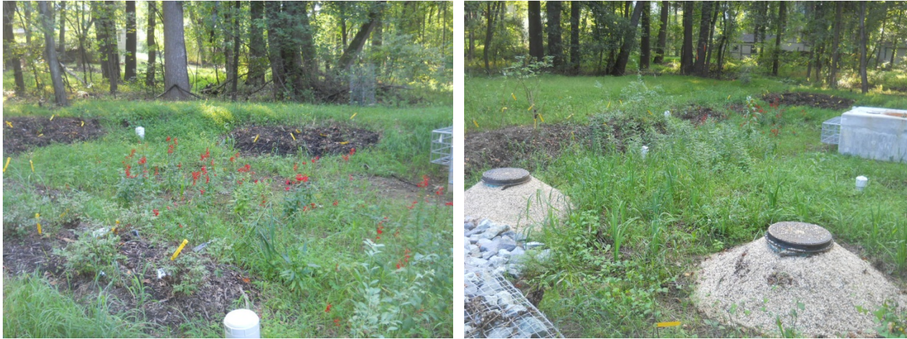
Figure 1-8: Submerged Gravel Wetland in Silver Spring, Montgomery County, MD
