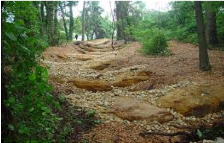
Figure 1-17: Regenerative Step Pool System Conveyance in Anne Arundel County
