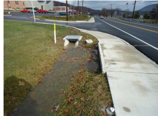
Figure 1-6: Grass Swale Example along MD 220 in Washington County
