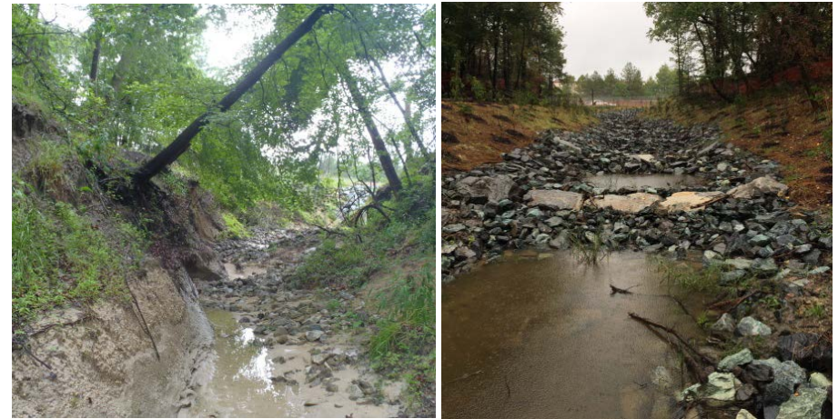
Figure 1-18: I-97 Outfall Before and After Stabilization in Anne Arundel County
