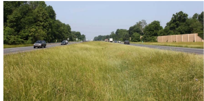
Figure 1-4: Existing Grass Channel along Median of I-70 in Baltimore County
