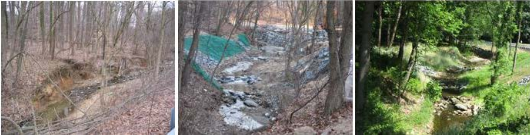
Figure 1-16: SHA Stream Restoration Project at MD 139 Before, During, and After Construction
