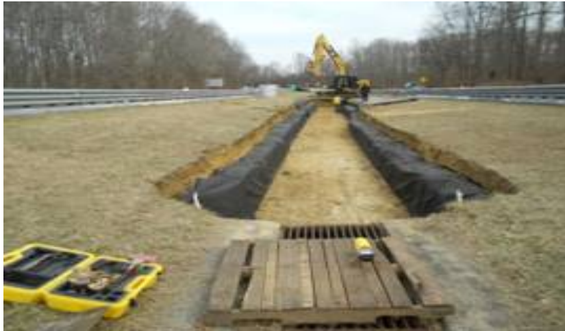
Figure 1-7: Bio-Swale during construction along MD 214 in Prince George's County
