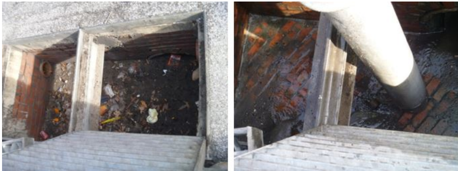
Figure 1-20 – Inlet Catch Basin Cleaning Before and After
