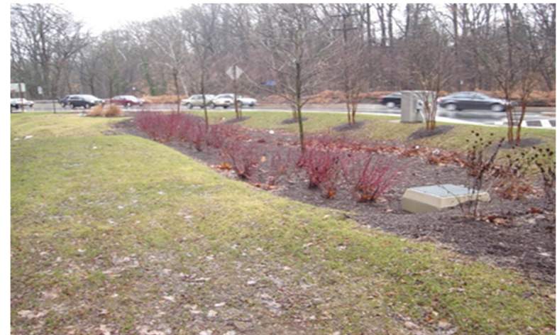
Figure 1-10: Bioretention Facility at MD 139 in Baltimore County
