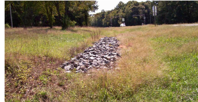
Figure 1-11: Infiltration Trench along US 113 in Worcester County
