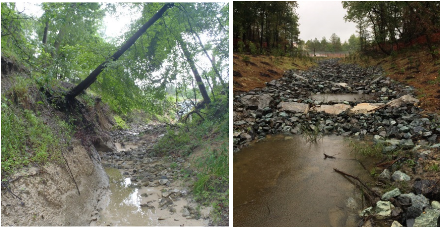
Figure 1-18: I-97 Outfall Before and After Stabilization in Anne Arundel County
