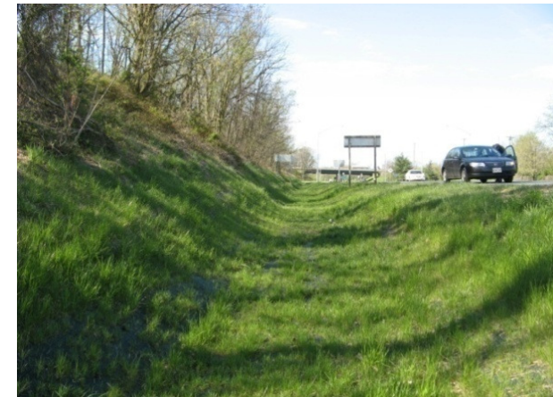
Figure 1-13: Before and After image of a Concrete Ditch Removal along I-70 in Washington County
