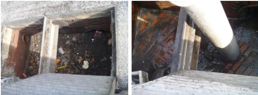
Figure 1-20 – Inlet Catch Basin Cleaning Before and After
