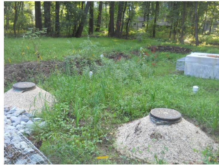
Figure 1-8: Submerged Gravel Wetland in Silver Spring, Montgomery County, MD
