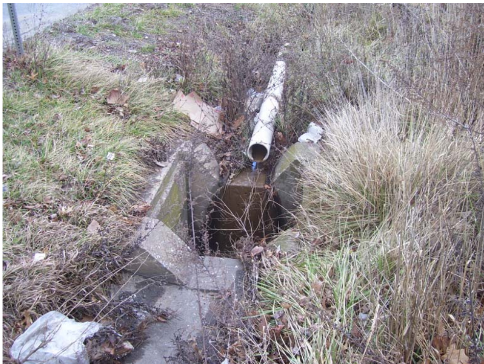
PVC pipe discharging to SHA inlet along MD140.
