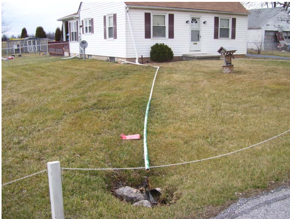
PVC pipe discharging to SHA drainage at 6155 Taneytown Pike.
