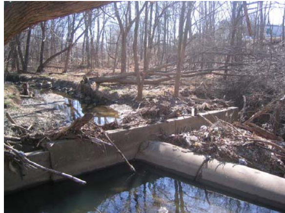
Dam with Upstream Debris and Sediment
