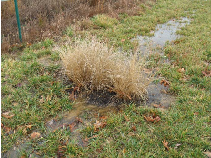
Figure 3-6. Close up of Vegetated Check Dams on MDE Swale, Maryland Route 32 (after storm event) (December 2007).
