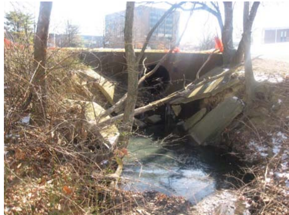
Failing Infrastructure and Outfalls within Degrading Reach of LDB
