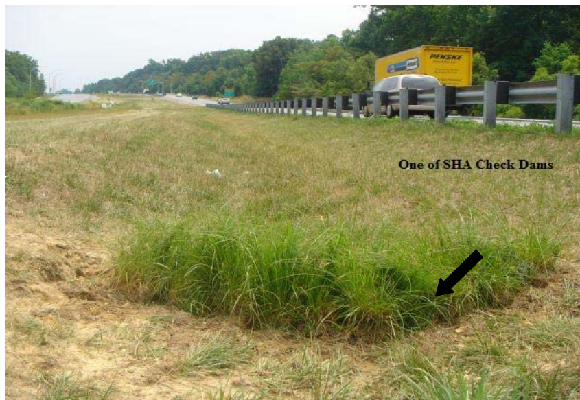
Figure 3-4. Vegetated Check Dams on SHA Swale, Maryland Route 32 (August 2007)
