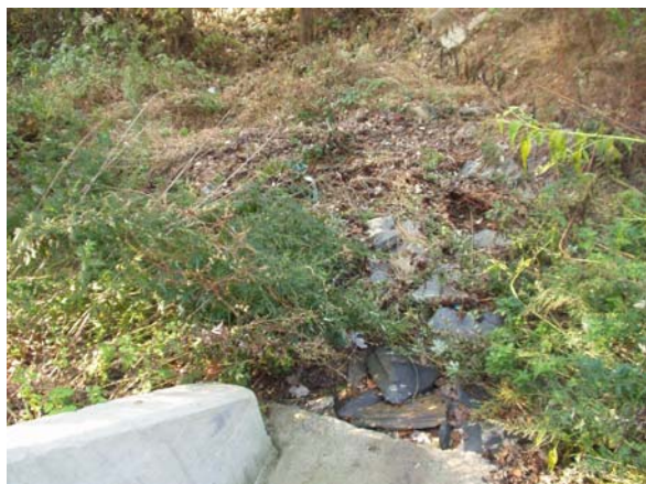
Failed Outfall at Site 43 in Harford County
