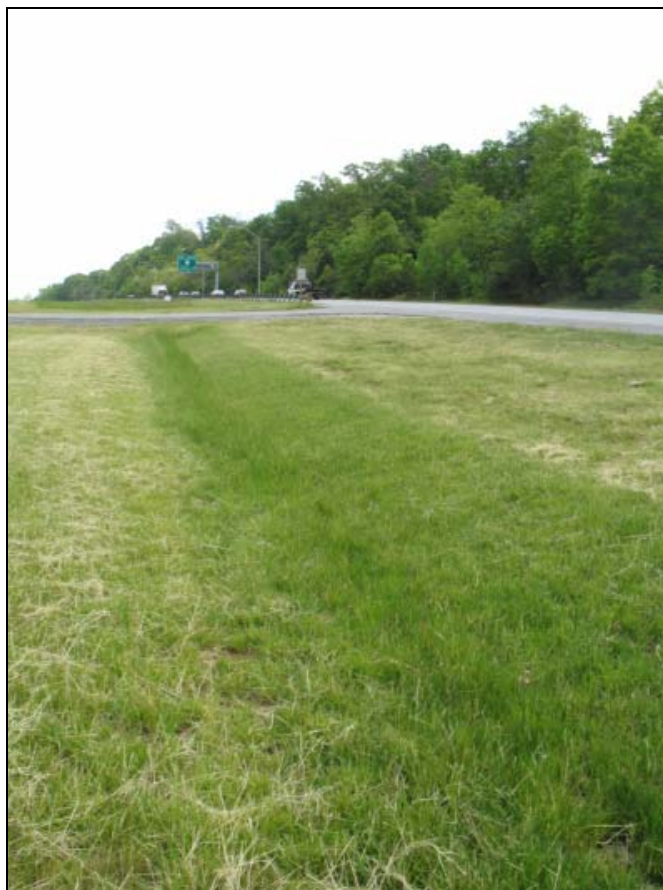
Figure 1. Grass swale with filter strip located on Maryland Route 32
