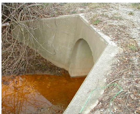
Examples of iron flocculant
