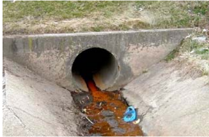
Examples of endwall structures
