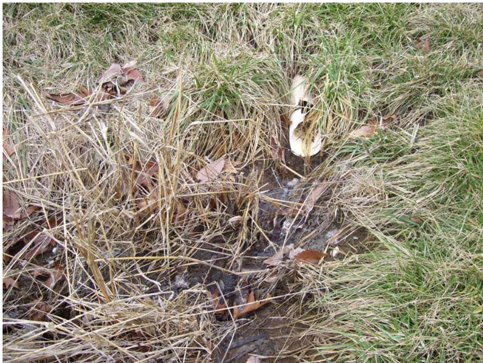
PVC pipe discharging to SHA culvert at 1709 Manchester Road.
