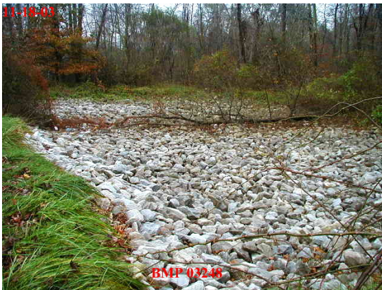
Figure 3-6 Infiltration Trench Investigation / Remediation Project along MD 43 – sites targeted for enhancement and retrofit
