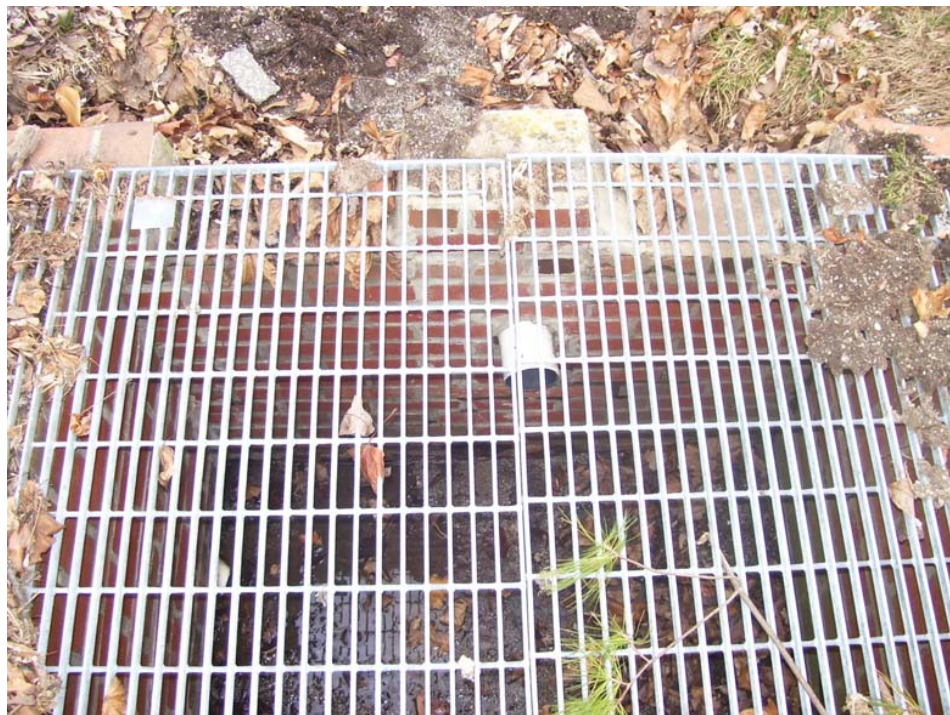
PVC pipe discharging to SHA inlet, at 1836 Taneytown Pike.
