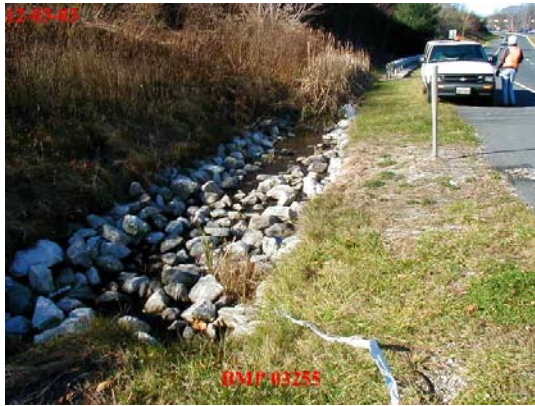
Figure 3-5 Infiltration Trench Investigation along MD 43 – sites to be replace in kind
