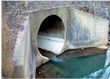
Examples of endwall structures
