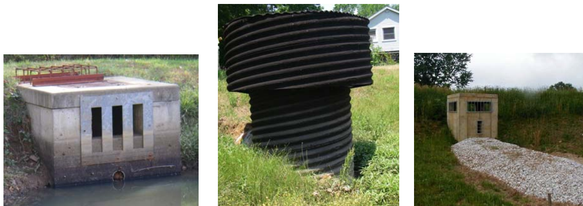
Example of riser structure in stormwater BMPs
