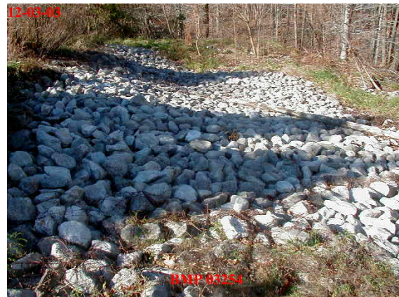
Figure 3-6 Infiltration Trench Investigation / Remediation Project along MD 43 – sites targeted for enhancement and retrofit
