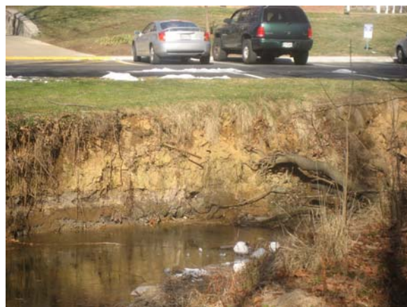
Development Encroachment Limits Access for Flood Flows and Results in Bank Erosion
