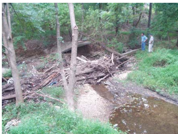
Debris and Sediment Upstream of Dam
