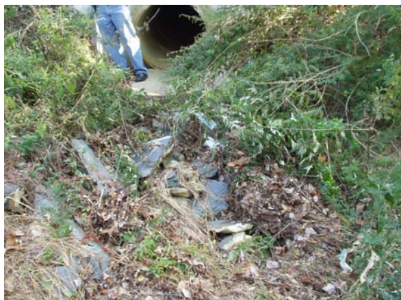
Failed Pipe Outfall at Site 43 in Harford County
