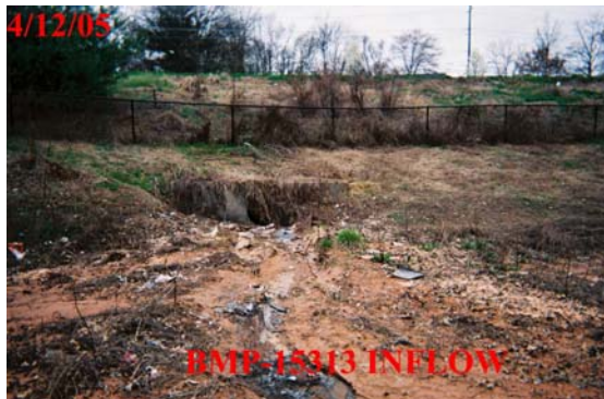
Figure 3-2: BMP15313 - Significant Inflow and Accumulation of Sediments and Debris
