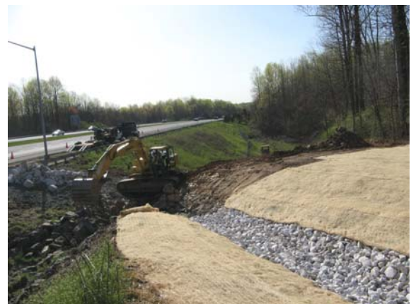
Figure 3-3: Inflow Channel Stabilization (BMP13007) - during construction
