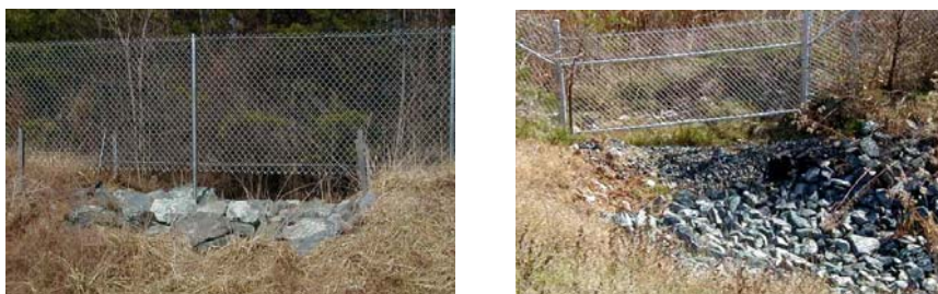
Example of emergency spillways
