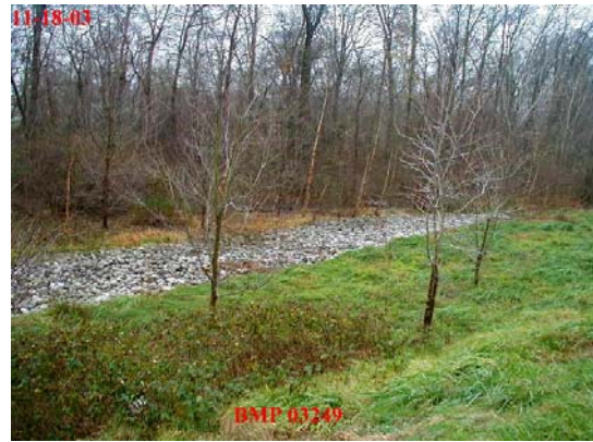
Figure 3-5 Infiltration Trench Investigation along MD 43 – sites to be replace in kind
