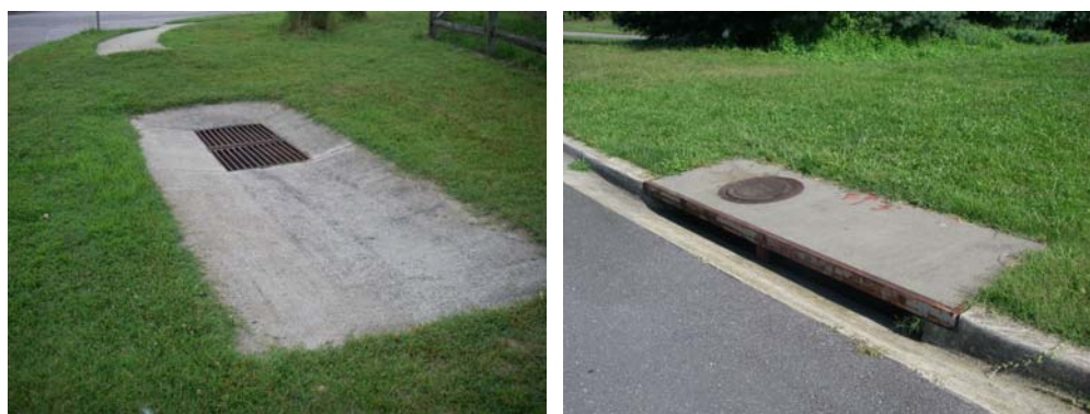
Example of inlet structures
