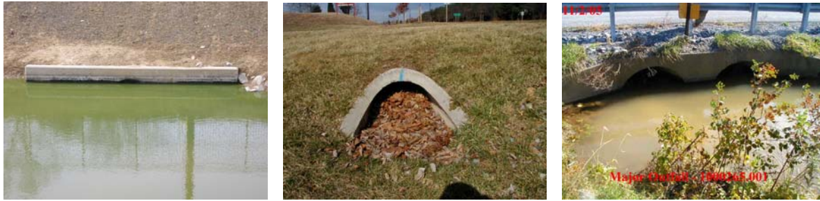
Examples of structures that would receive a “2” value for structure issues, such as submerged structures or structures with minor accumulation of debris and sediment.
